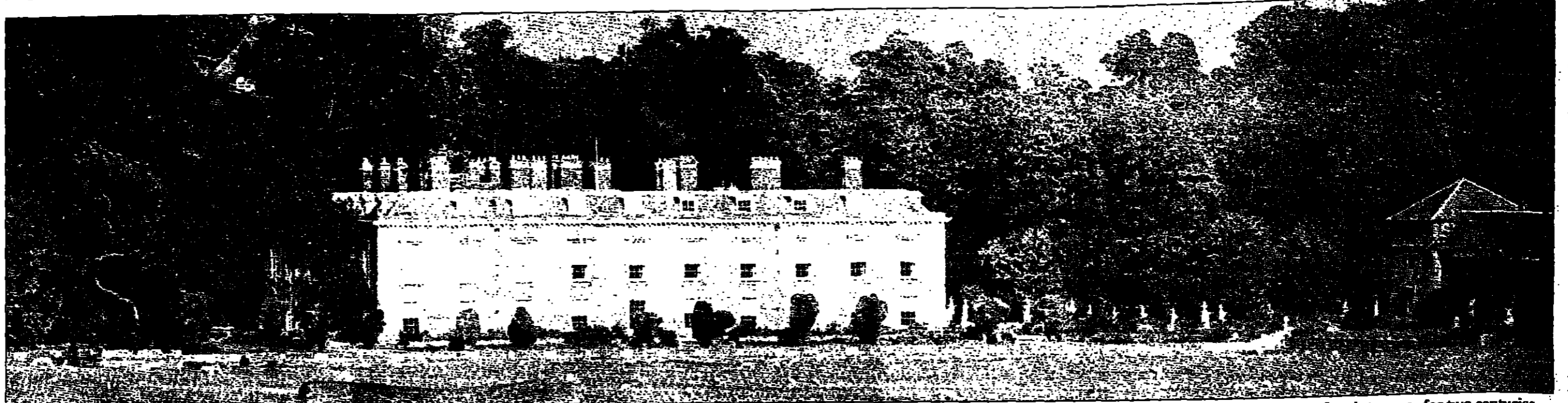
The austere exterior of Althorp House has never been called beautiful: yet in a practical sense, Henry Holland's work has helped the outward appearance of the house survive with the minimum of maintenance for two centuries
